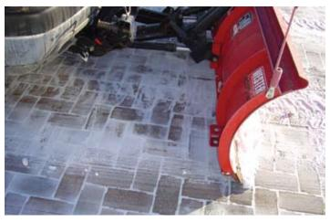
Figure 9. PICP is snow plowed like any other pavement.
